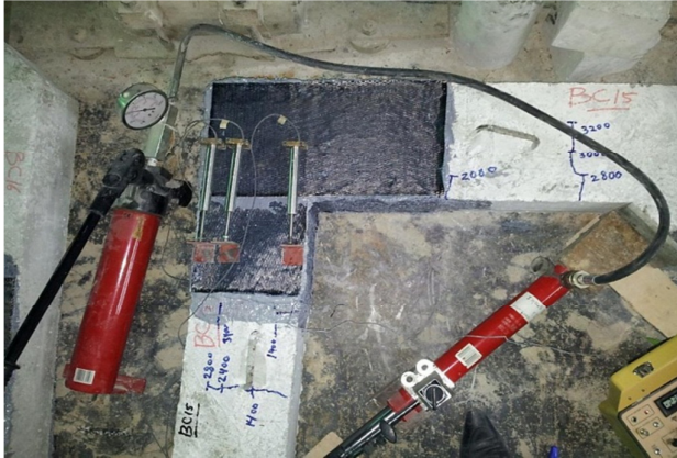
Fig.(7) Crack pattern of the specimen preloaded until first crack load and strengthened with full-CFRP (BC15)
